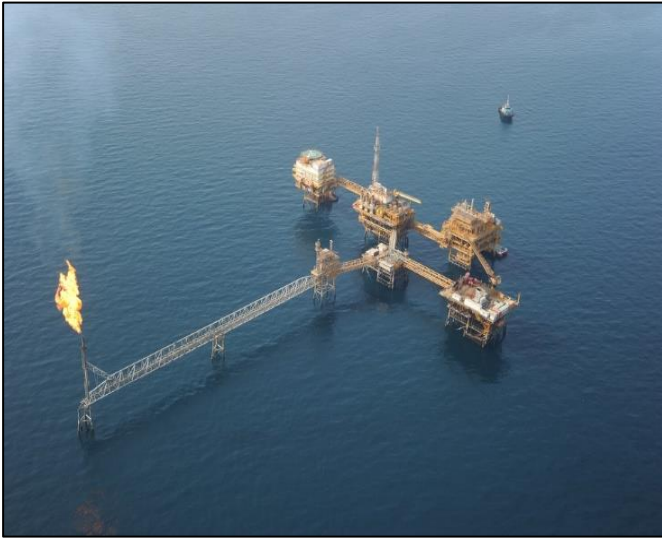
Figure 1: Foroozan oil complex [28]
