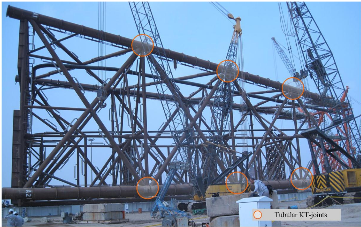
(a) Tubular KT-joints in a jacket structure during the fabrication
