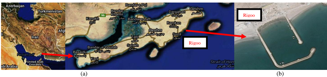
Fig. 2) a) Location of Rigoo Harbor and b) Aerial view of the study breakwater
